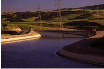
SOURCE WATER PUMPING (WSO)
