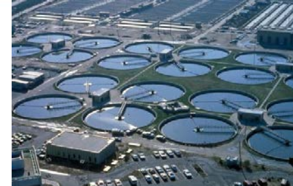
WASTEWATER TREATMENT (WWTP)
