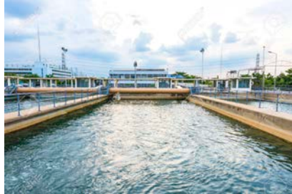
WATER TREATMENT (WTP)
