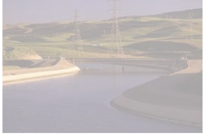
SOURCE WATER PUMPING (WSO)
