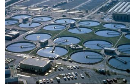
WASTEWATER TREATMENT (WWTP)
