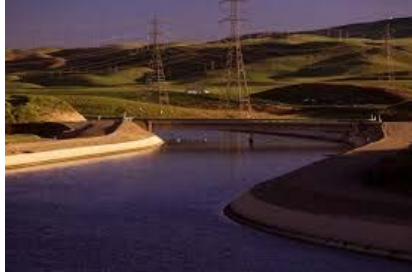
SOURCE WATER PUMPING (WSO)
